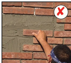
Thin-set brick or stone is an unacceptable substitute material for brick and stone.
