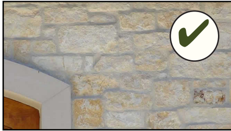
Rough stone laid in a random-ashlar pattern is appropriate for the Historic District.
