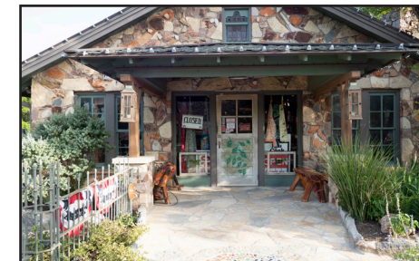
Giraffe style masonry with unique materials is a key characteristic of buildings in Wimberley.
