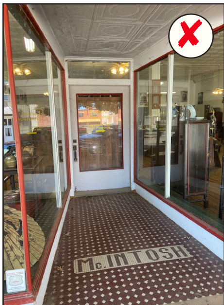
Deeply recessed storefront entrances are not appropriate.
