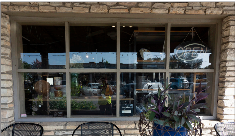
Typical storefront windows in the Historic District are wood-framed and have simple profiles.
