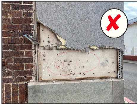
Covering historic masonry can cause damage to the underlying historic material.
