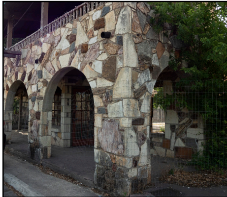
Giraffe-style masonry that includes a variety of masonry materials is a character-defining feature in Wimberley.
