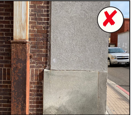
EIFS is an unacceptable substitute material for cast stone and stone.
