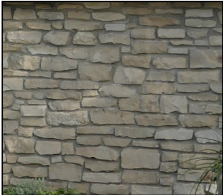
Many buildings have rough-faced limestone cladding in a random-ashlar pattern.
