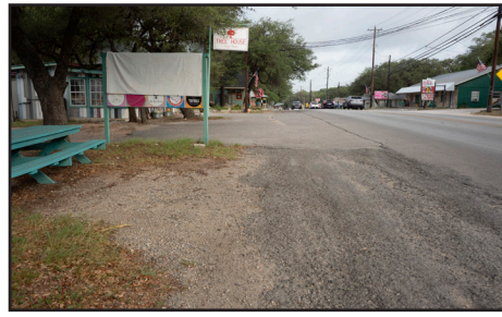
Many streets outside the Square lack sidewalks.
