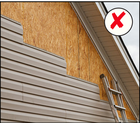
Vinyl siding is an unacceptable substitute material for wood siding.
