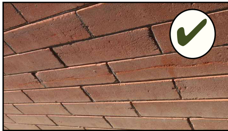
Repoint missing or deteriorated joints with an appropriate, compatible mortar.
