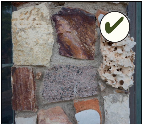
Giraffe-style masonry that includes a variety of masonry materials is appropriate for Wimberley.
