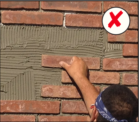
Thin-set brick or stone is an unacceptable substitute material for brick and stone.
