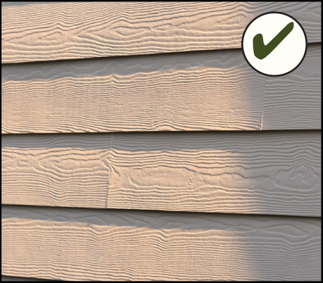
Cementitious board siding is an acceptable substitute for a wood siding, as long as the profiles are similar.
