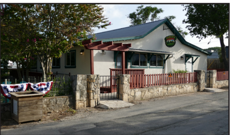
Buildings in the Square have shallow setbacks.
