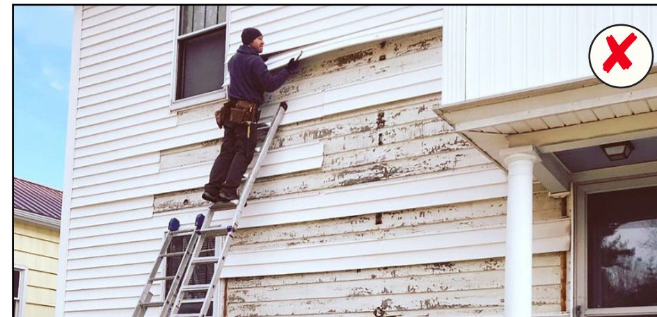
Damaged materials should be repaired or replaced in-kind instead of covered with an inappropriate substitute material.
