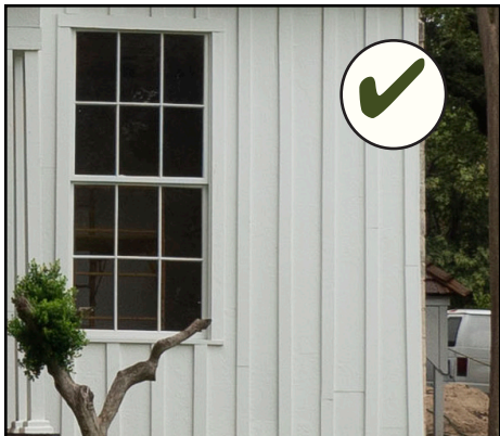
Board-and-batten wood siding is appropriate for certain architectural styles in Wimberley.
