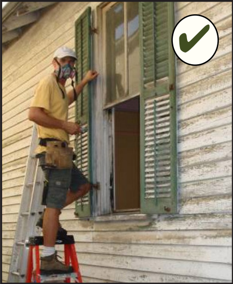
Maintain existing paint coatings on exterior wood to prevent exposure to wind, sun, and rain.
