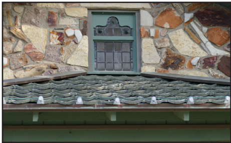
Exposed rafter tails and low-pitched roofs are a characteristic of the Craftsman style.
