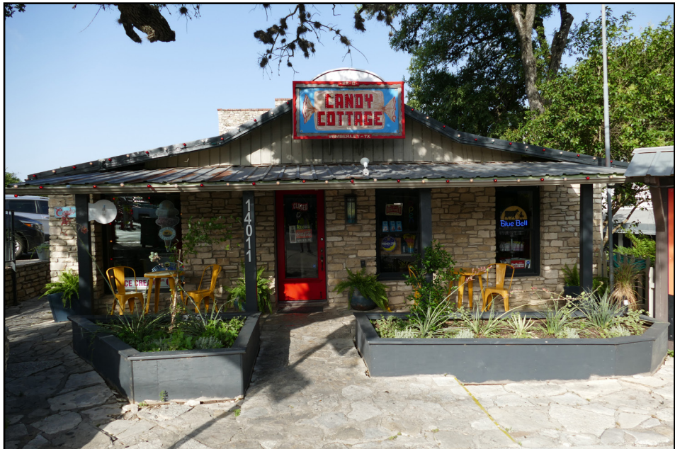
Each architectural style has different character-defining features. The character-defining features of this Vernacular-style building include limestone and giraffe-style masonry, board and batten siding on the gable, and wood windows.
