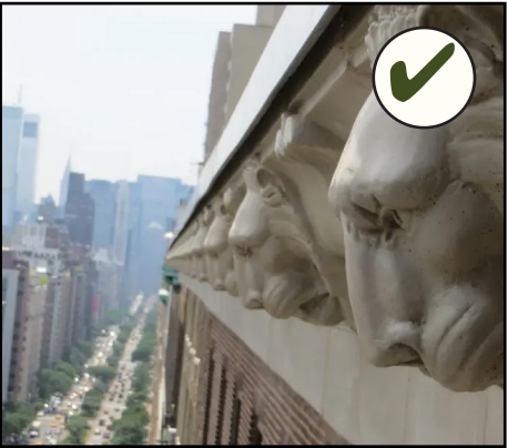
A fiberglass cornice is an acceptable substitute for a formed metal cornice.
