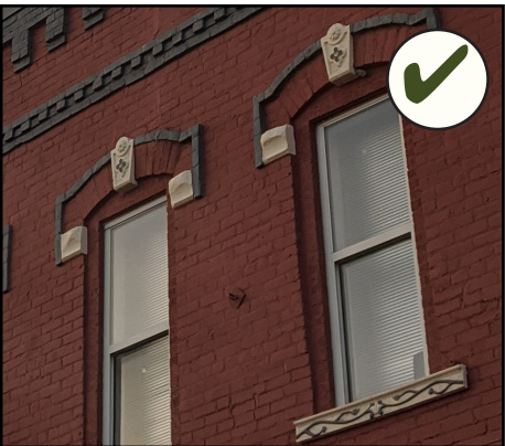
Metal clad wood windows with historic profiles are an acceptable substitute for upper-story wood windows.
