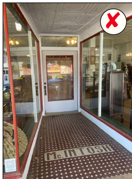
Deeply recessed storefront entrances are not appropriate.
