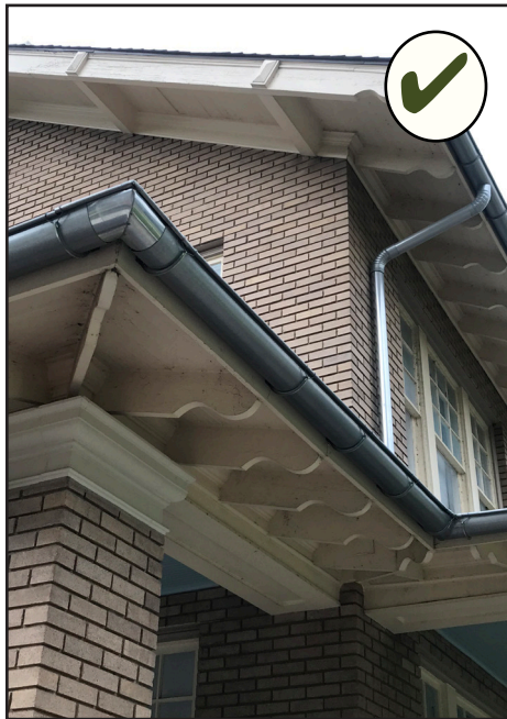
Regularly clean gutters and downspouts.
