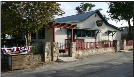
Buildings in the Square have shallow setbacks.
