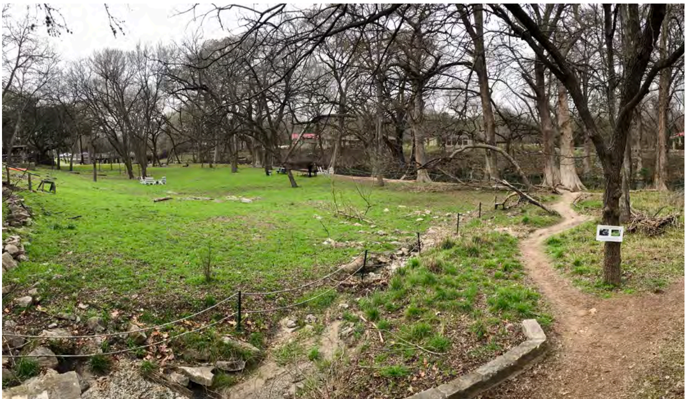
Outfall #1 - Erosion and Fencing, Winter 2019
